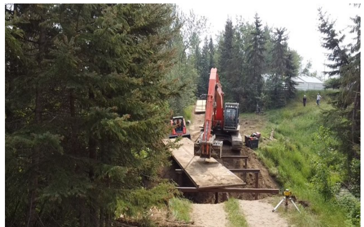
Lower Peace Creek Crossing Installation Project
